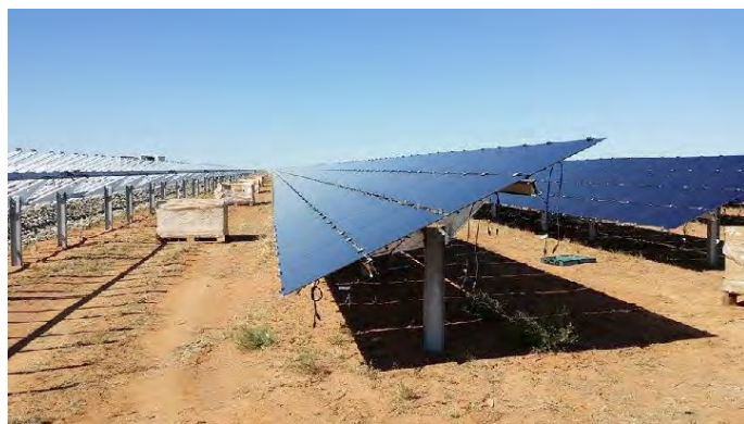
Image from Australian Renewable Energy Agency
