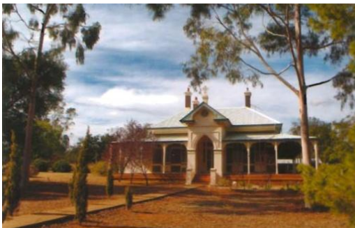
Parish house, Ardlethan
